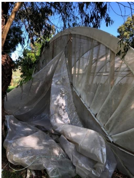
Fig. 3 Damaged Solarweave cover after the wind storm.
