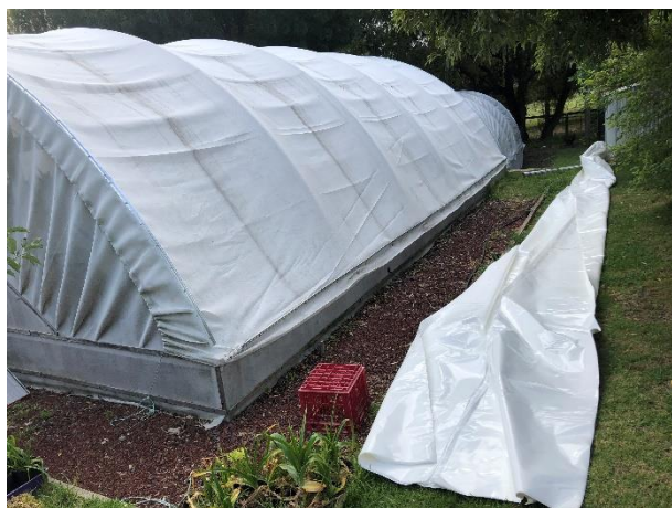
Fig. 6 Aluminium strips in place ready for the film.
