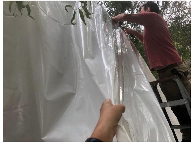
Fig. 9 Pulling the film taut.
