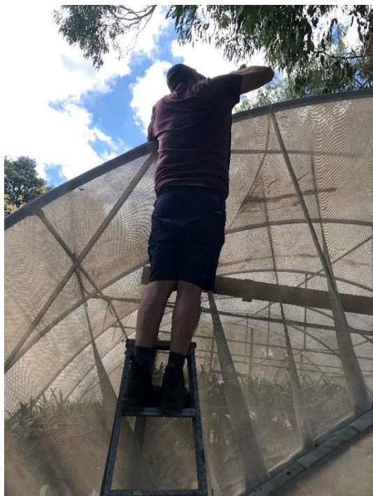
Fig. 5 Attaching the aluminium clipping strip over the hoop
