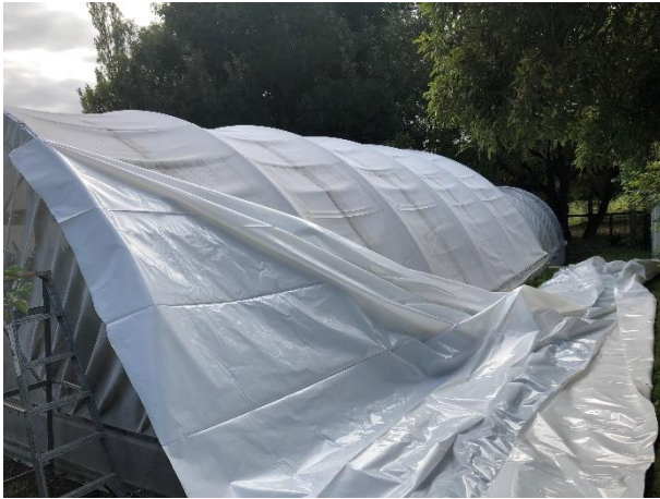
Fig. 7 Pulling and clamping one side at a time.
