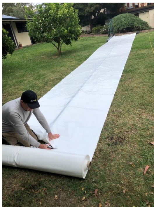
Fig. 4 Cutting the correct length with scissors.
