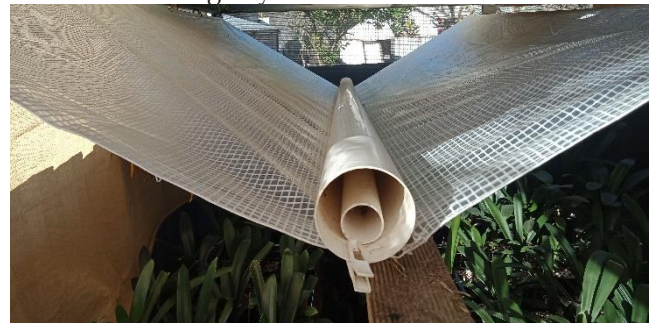
Fig. 20 Storm water pipe in gully of clear tarp
