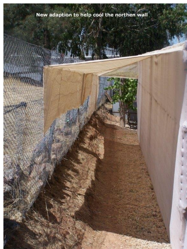
Figure 8 - New adaption to help cool the northern wall
